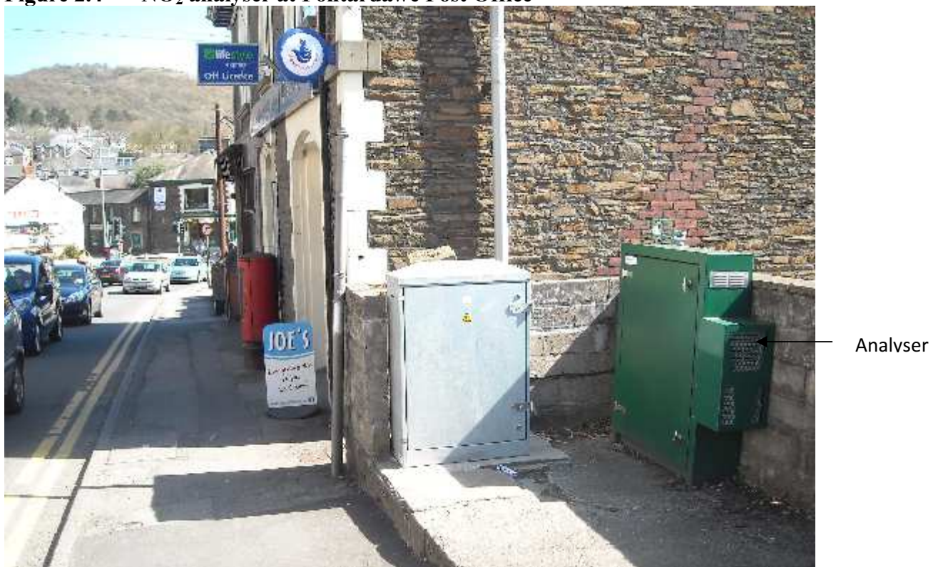
Figure 2.4 NO 2 analyser at Pontardawe Post Office
